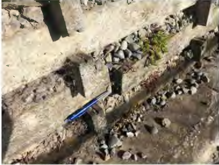
Deformation of timber crib retaining wall.
