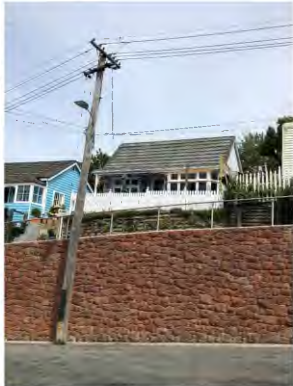
Figure 2 – Photo of street side retaining wall to front of property. Timber crib retaining wall set back approximately 2 metres from stone-faced wall, with dwelling set back an additional 2.2 metres.
