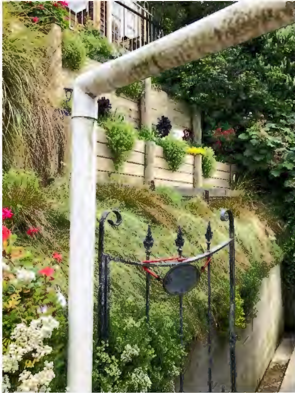
Figure 3 – Photo of stepped retaining walls at rear of dwelling
