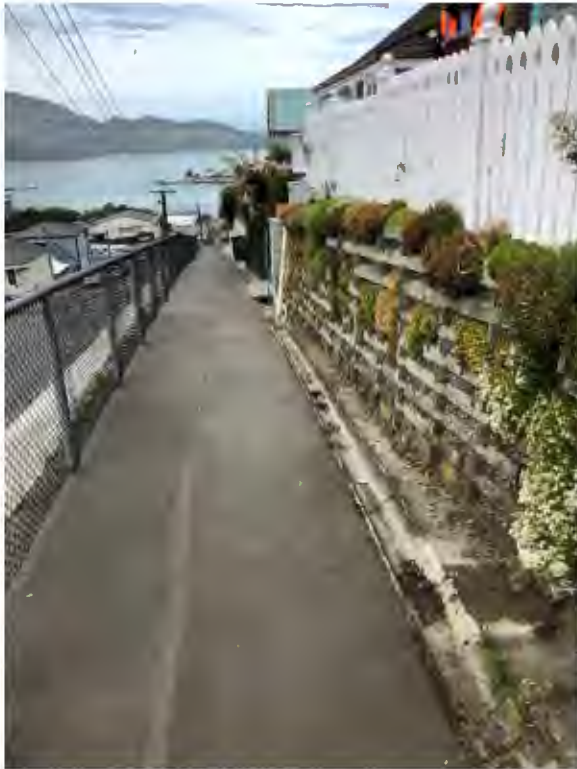
Figure 1 – 1.2 m -1.5 m timber crib retaining wall located at front of property.
